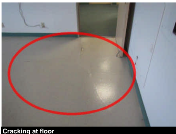
Cracking at floor
