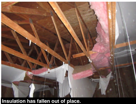
Insulation has fallen out of place.
